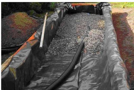
A larger system will need a pipe within the reservoir to help fill it. "Ag pipe" is fine for this job. Shade cloth or geotextile goes over the gravel, then soil.
